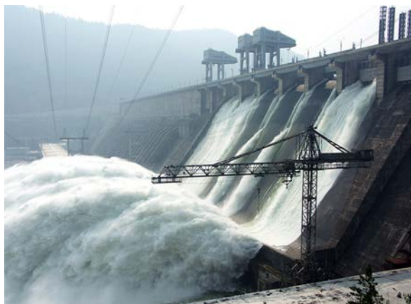
Figure 7.38 Hydroelectric facility (credit: Denis Belevich, Wikimedia Commons)
